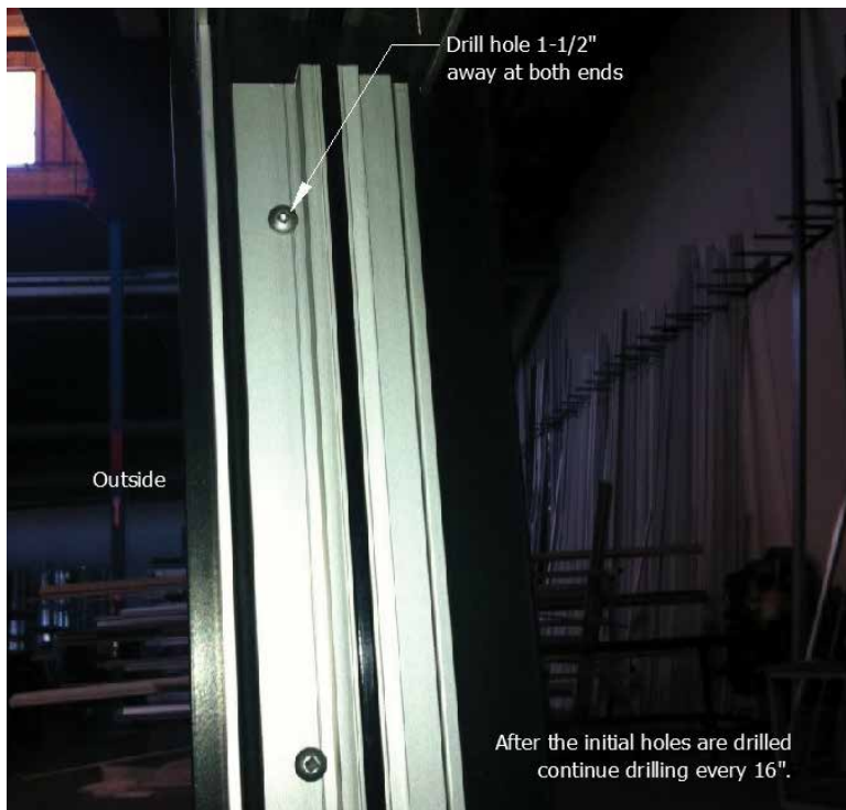
DISTANCE MEASURED FOR JAMBS
